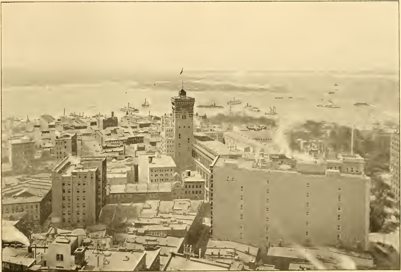
VIEW LOOKING SOUTH FROM ROOF OF OFFICE BUILDING, 66 BROADWAY
