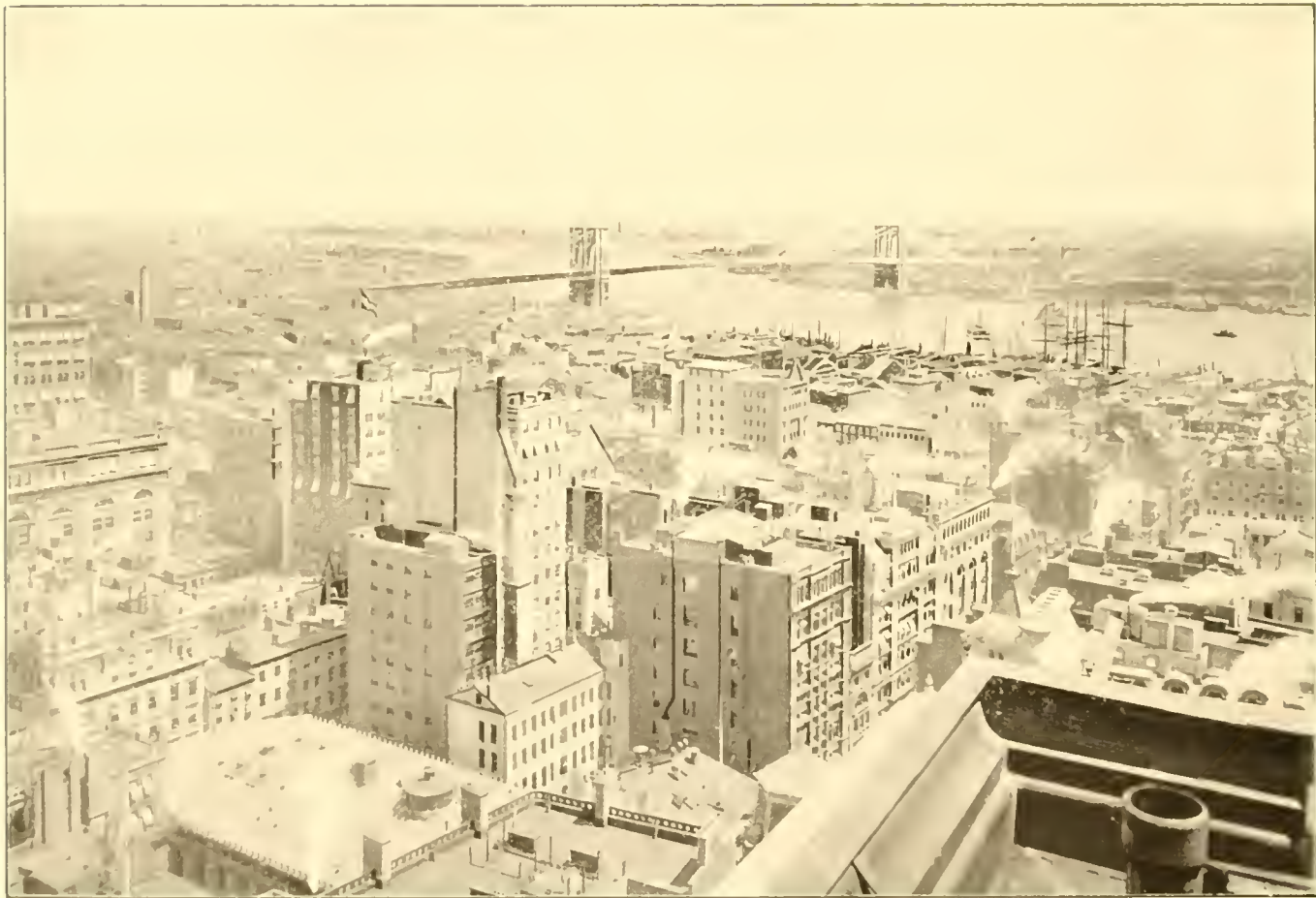
VIEW LOOKING NORTHEAST FROM ROOF OF OFFICE BUILDING 60 BROADWAY
