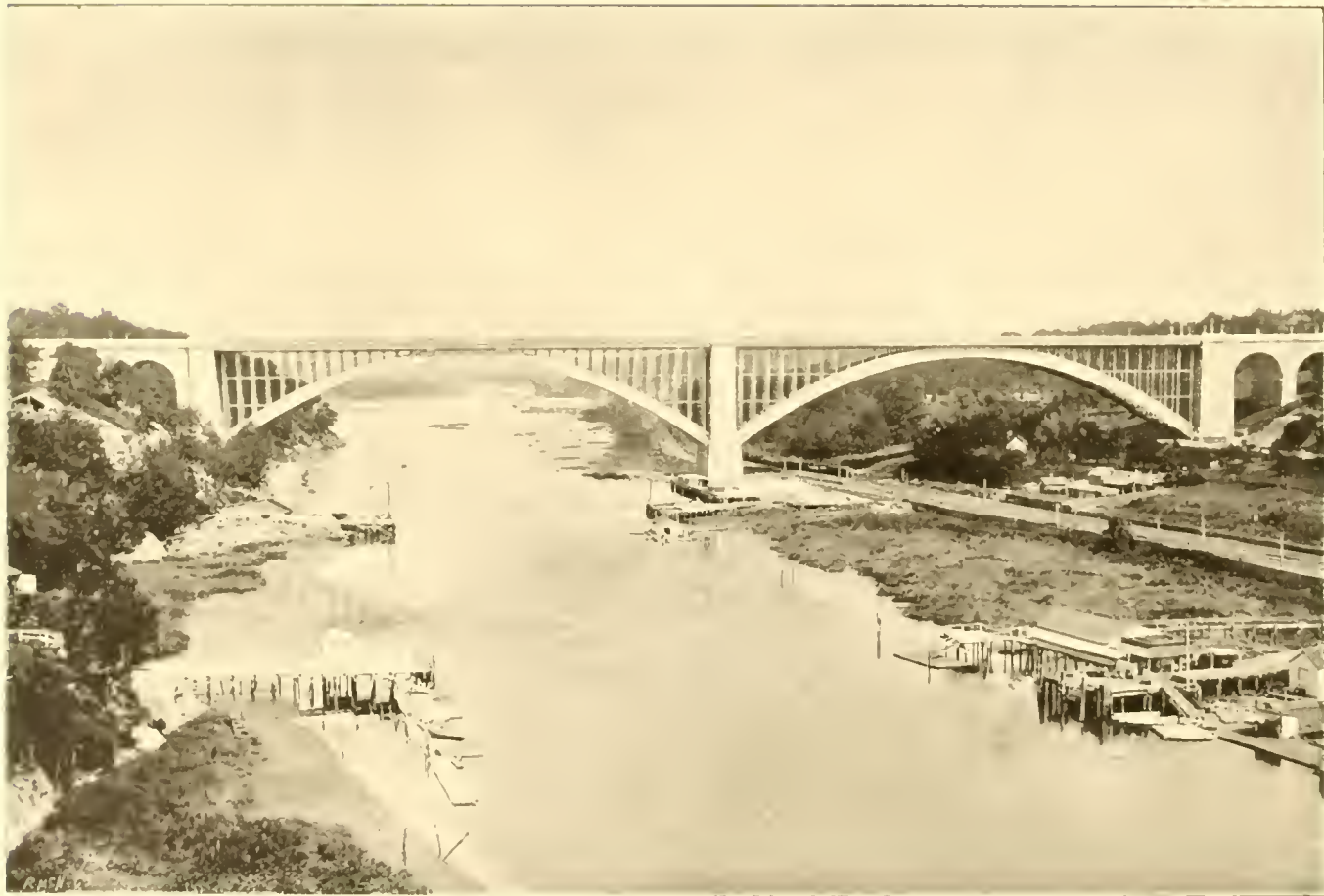
THE WASHINGTON BRIDGE ACROSS HARLEM RIVER From One Hundred and Eighty-first Street and Tenth Avenue to Aqueduct Avenue
