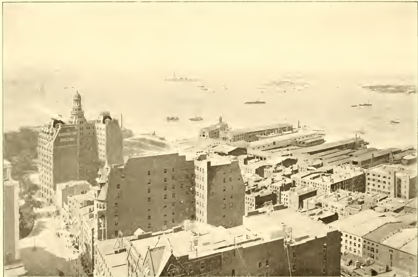
VIEW LOOKING SOUTHWEST FROM ROOF OF OFFICE BUILDING, 66 BROADWAY.
